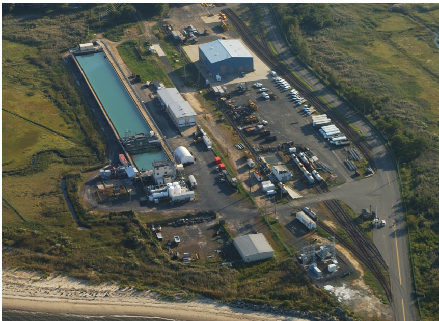
FIGURE 3-9 Aerial view of the OHMSETT test tank facility.
